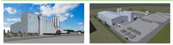
The 4.000  $m^2$  production hall will be built on a 40.000  $m^2$  site where the latest developed German machinery line will be installed for the production of 800.000  $m^2$  of paving stone per year.
